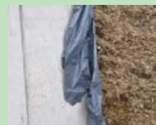
Lining the clamp walls with side sheets before filling the clamp is a key step to reducing air ingress.
